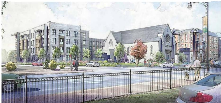
A new 230,000 square foot four-story building over a one-story parking deck, will be connected to the existing structures and is designed to look like a series of separate buildings while providing a neighborhood feel.
